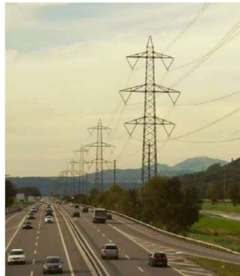
«tomorrow»: 5'600 MVA (Including GIL of 1700 MW)
